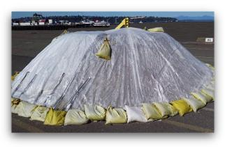
Protect stockpiles from wind and rain by using sandbags and tarps.
