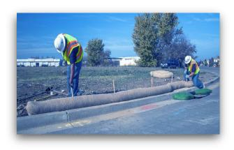
Protect exposed soil from erosion by using mulch, erosion blankets, or straw wattles.
