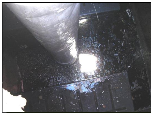
Removal of trash, sediment and debris.
