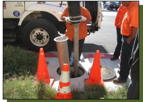
Insertion of vacuum hose into separation chamber.
